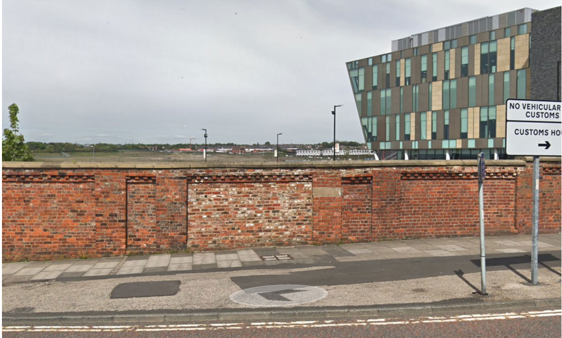
Figure 3 Former gateway through Mill Dam Wall
